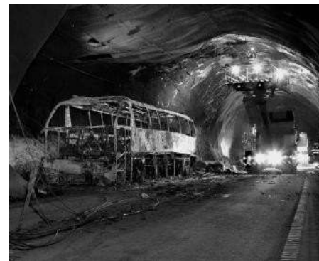
Gudvanga tunnel August 2015
