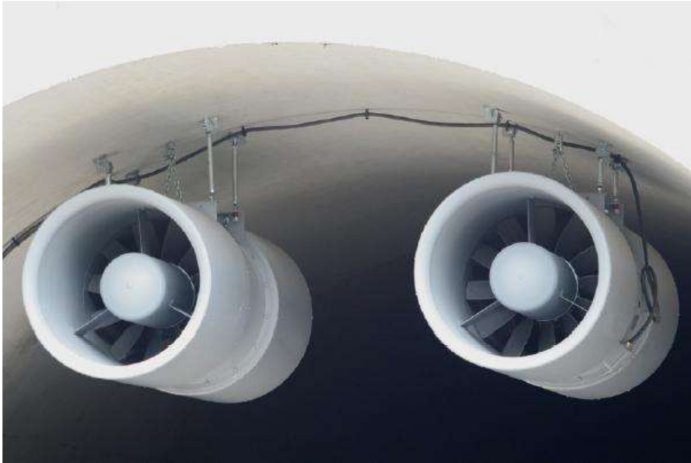
6 JET FANS (45KW each)
